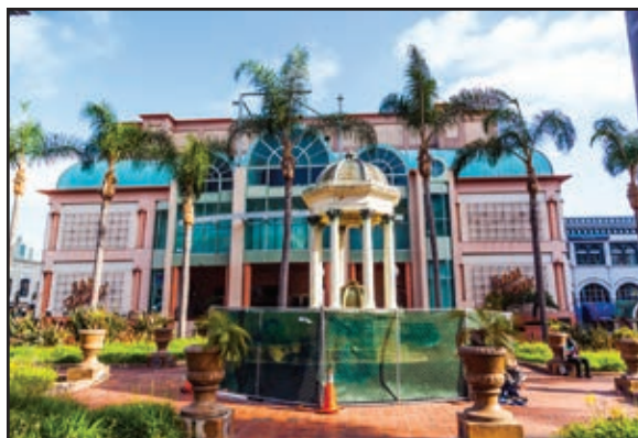
Facades of historic houses in the Gaslamp Quarter. Photo © Jorg Hackemann, Dreamstime.com.
